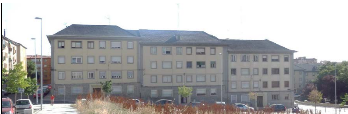
Figure 9. Current state of façade behind the block. Source: Author’s photo.
