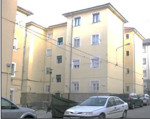
Figure 13. Current state of the first phase. Source: Author’s photo.
